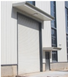
Electric rolling shutter door
