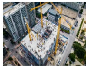
Steel structure building
