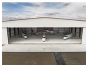
Steel structure garage/hangar
