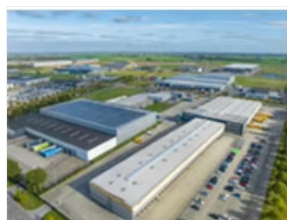
Steel structure warehouse
