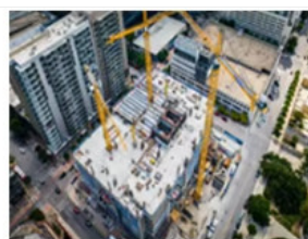
Steel structure building
