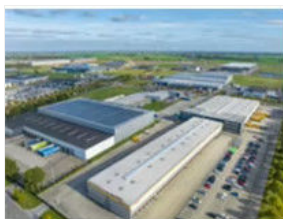
Steel structure warehouse
