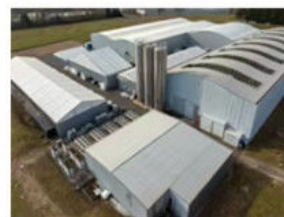
Steel structure livestock house
