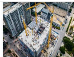
Steel structure building
