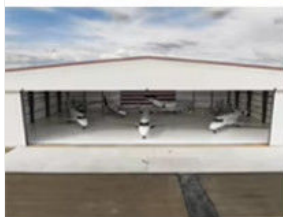
Steel structure garage/hangar
