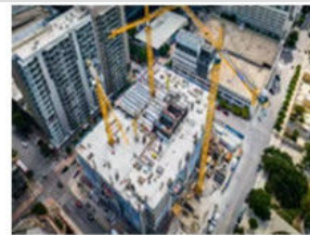
Steel structure building
