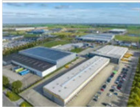
Steel structure warehouse
