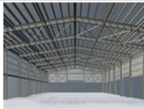
Steel structure factory building
