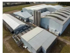
Steel structure livestock house
