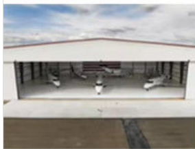
Steel structure garage/hangar
