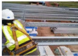
Install the Roof Purlin
