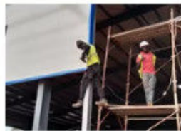
Install the Flashing Sheets
