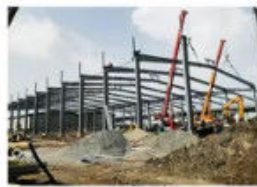
Install the Columns & Beams by Crane
