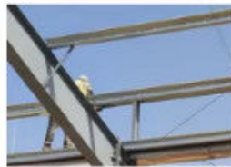
Install the Purlin Bracing
