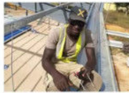
Install the Purlin Rod
