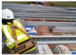
Install the Roof Purlin
