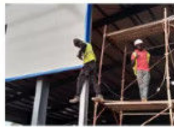
Install the Flasin Sheets
