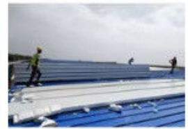
Install the Roof Panels
