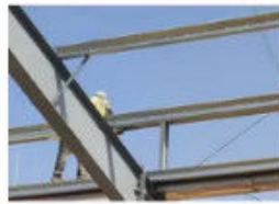
Install the Purlin Bracing
