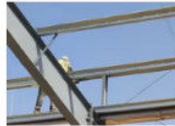
Install the Purlin Bracing
