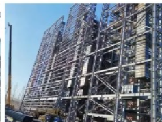
11. Steel structure construction finished effect
