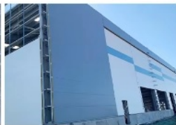
12. Exterior wall insulation system construction effect
