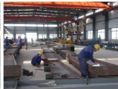
5. The steel plate was shot blasted to remove rust
