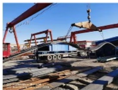
1. Choose steel plate, quality inspection after the start of the material
