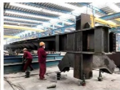
8. Inspect welded steel structure, prepare for galvanizing or painting
