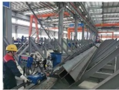
4. Drill holes into some steel plate parts
