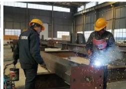
6. Start assembling the steel plate and spot welding it
