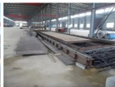
2. Distinguish the steel plate material, waiting for cutting
