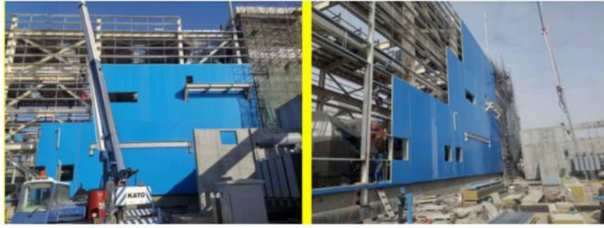
Gas Turbine Combined Cycle Power Station Expansion Project in Basra Iraq
