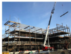
MULTI-STOREY BUILDING IN PHILIPPINES
