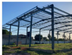
STEEL BUILDING IN ZIMBABWE
