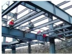
10. Spray paint and galvanize steel structure according to technical
