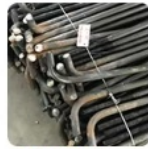
Embedded bolts for foundation
