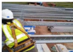
Install the Roof Purlin
