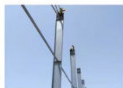
Install the Steel Rod
