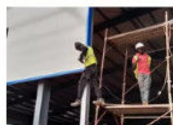
Install the Flashing Sheets
