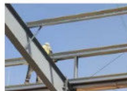
Install the Purlin Bracing
