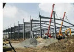
Install the Columns & Beams by Crane
