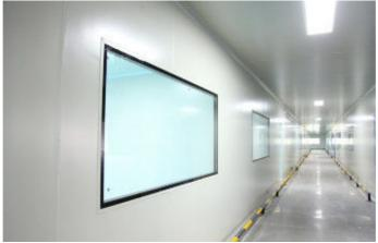
To further expand these viewing points and make our clean rooms even more "open" and bright, we have created glass panels, one or two meters in height, for uninterrupted continuous vision. The glass panels are always produced with 45 mm thick double glazing completely flush with the surface of the partition walls or doors.
