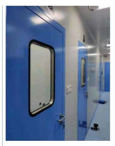
The clean room doors are made of aluminium frame; the panel is made with the same sandwich as the partition walls, allowing total flush-fitting between the components and the wall itself.
