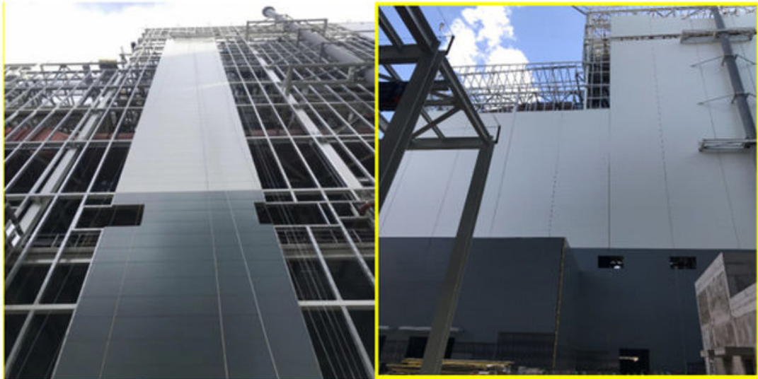
2 * 1000MW Supercritical Power Plant Phase III Expansion Project in China
