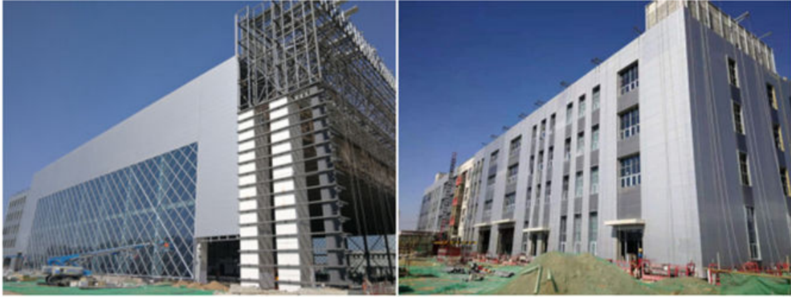
East Airlines Maintenance Area of Beijing New Airport
